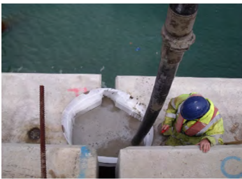
Figure 28—Shear Key
