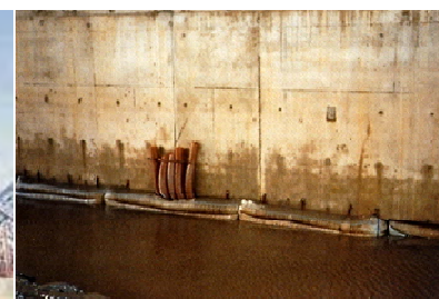
Figure 18 – Grout Bag Foundations
