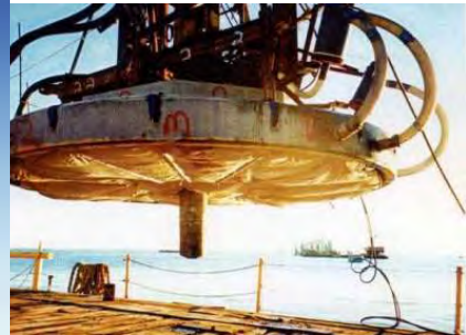
Figure 21 – Initial Pad, Forms Condensed
