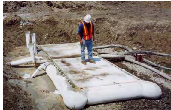
Figure 25 – Grout Bag Trials
