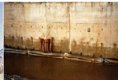
Figure 18 – Grout Bag Foundations
