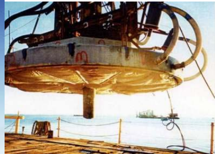
Figure 21 – Initial Pad, Forms Condensed
