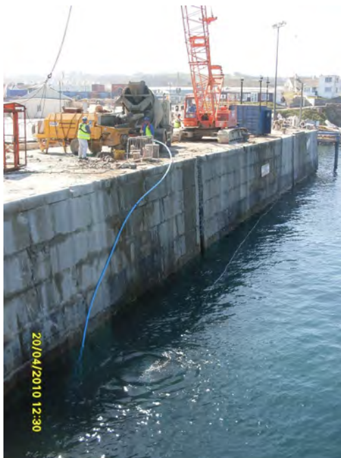
Mattress filling from Commercial Quay
