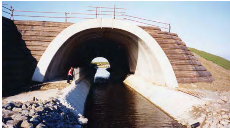
Culvert and Channel Construction
