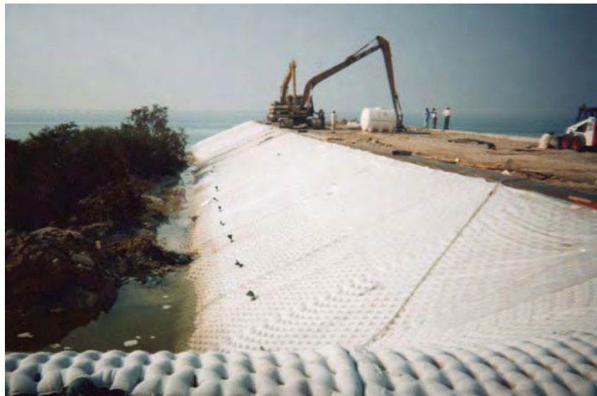
Laid & Filled Mattress Along Embankment
