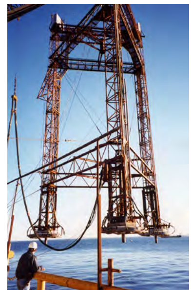
Hard Pad Installation Frame
