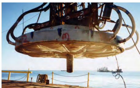
Pad Showing Fixed Fabric Form Ready for Positioning
