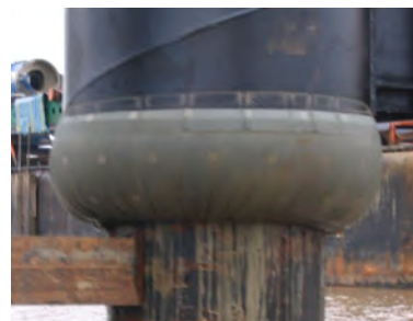
Fender Pile Seals
