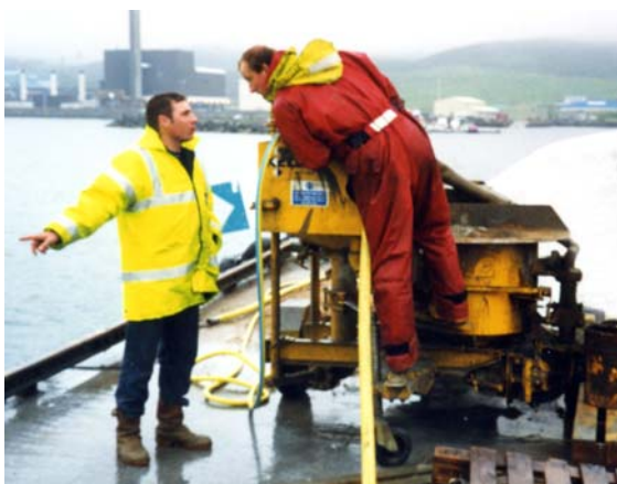
Micro Concrete Mixing and Pumping
